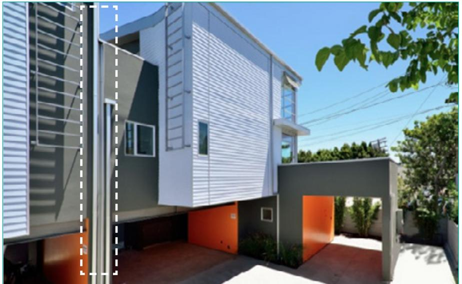
Structural Independence - Flashing detail over two separate walls (dashed line).
