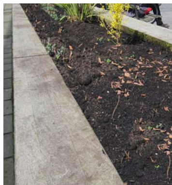
Figure 29. Removing the planter edge so that it is flush with surrounding impervious surfaces allows stormwater runoff to irrigate the garden
