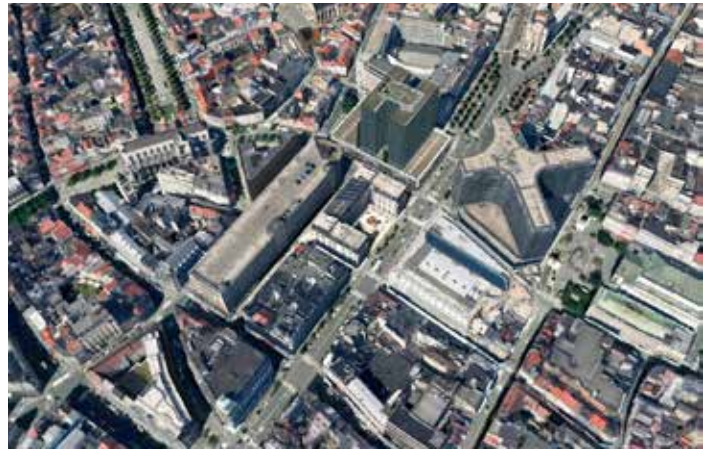
Figure #6. Existing Roof Conditions Brussels, Belgium Adapted from Google Earth Image
